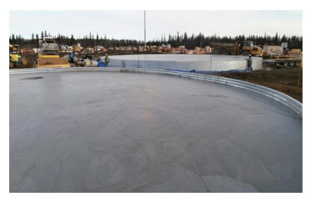
The use of corrugated steel panels is an effective and cost-saving technique for the construction of gravel filled or concrete filled foundation rings
